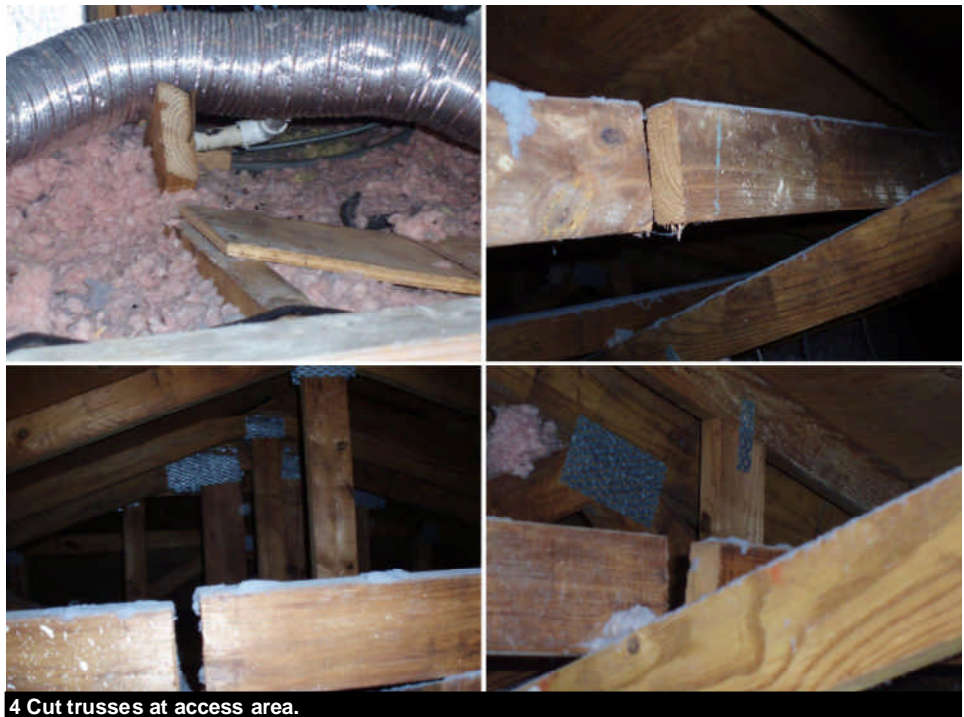
4 Cut trusses at access area.
