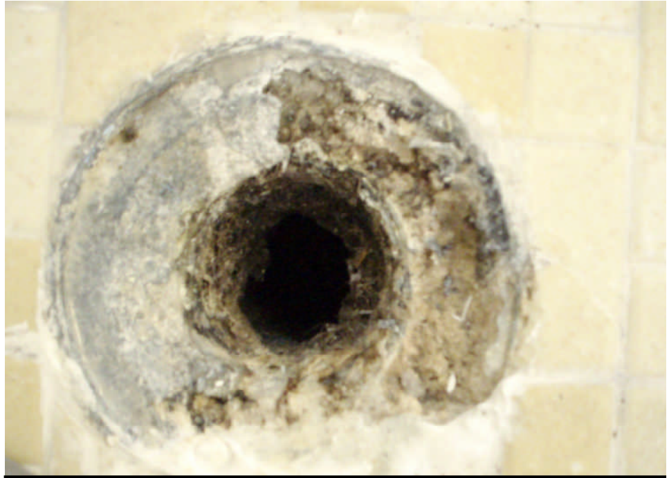
Damaged drain.
