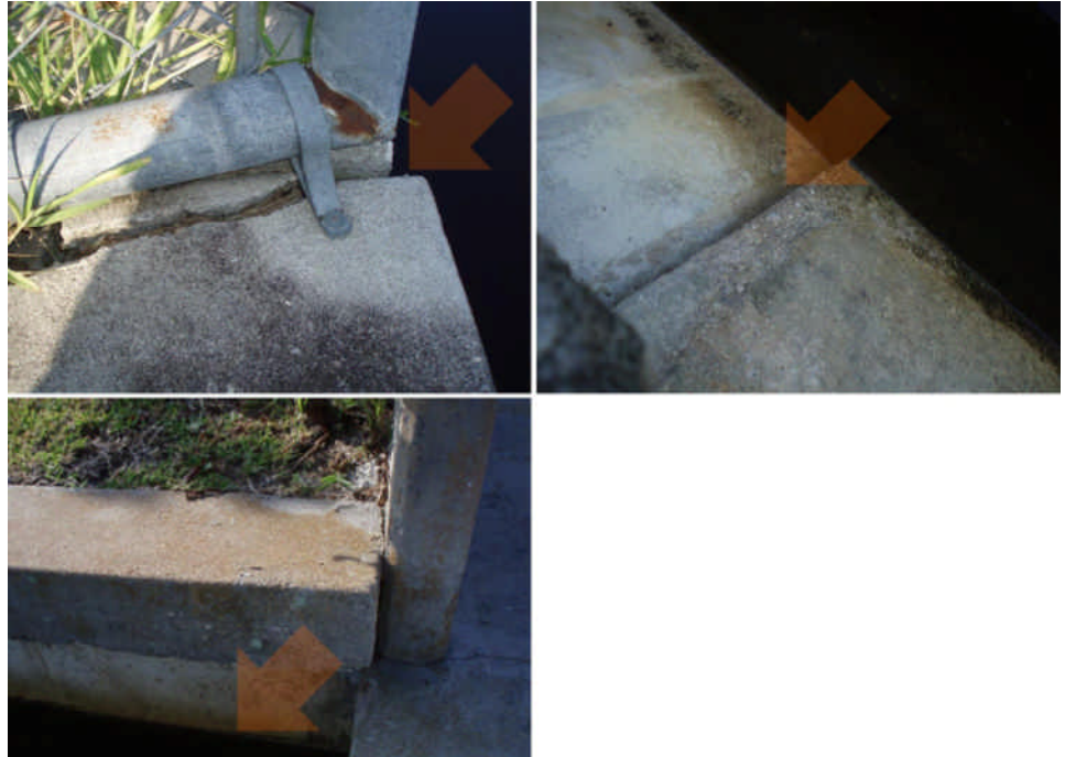
Movement in wall. High Water.
